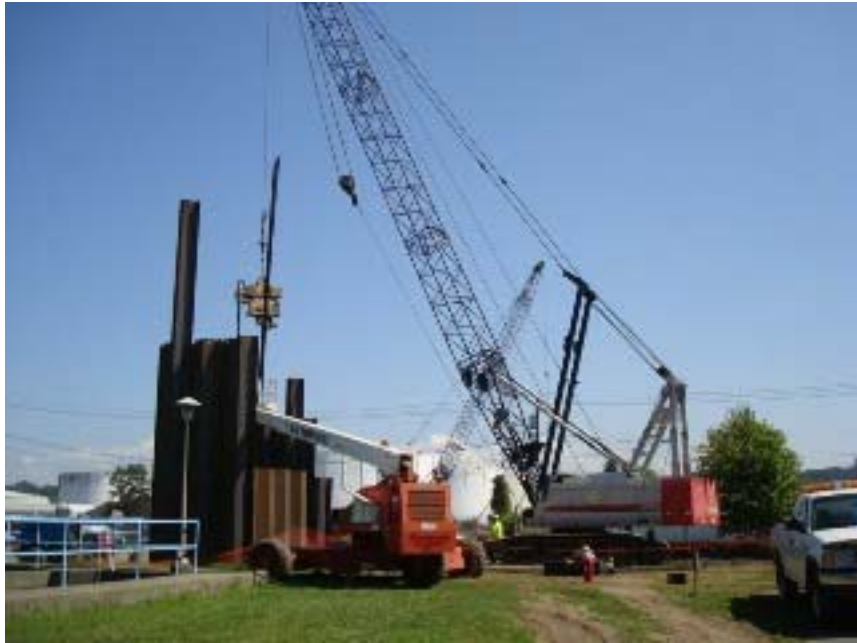
Diversion Chamber Construction at South Plant
