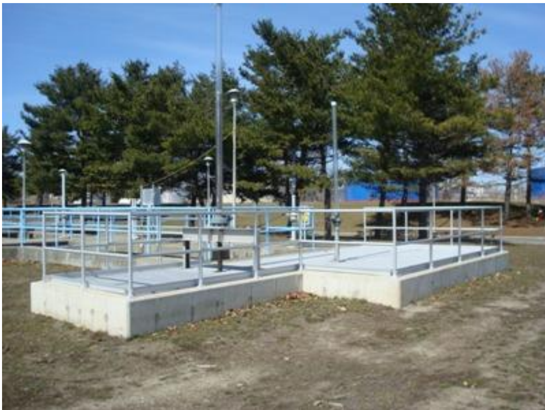
Gray Water Diversion Chamber
